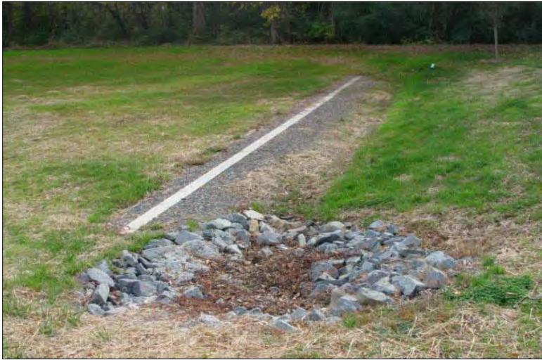
Figure B-37: Grass Filter Strip with Upstream Level Spreader (NCSU BAE, 2011)
