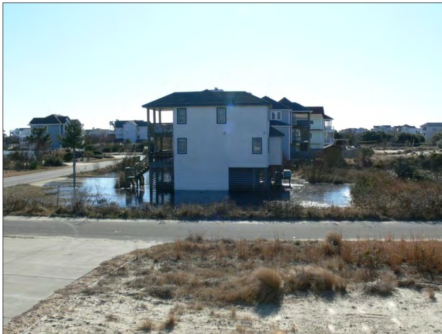
Figure 2-10: Fill on Surrounding Lots Exacerbates Flooding
