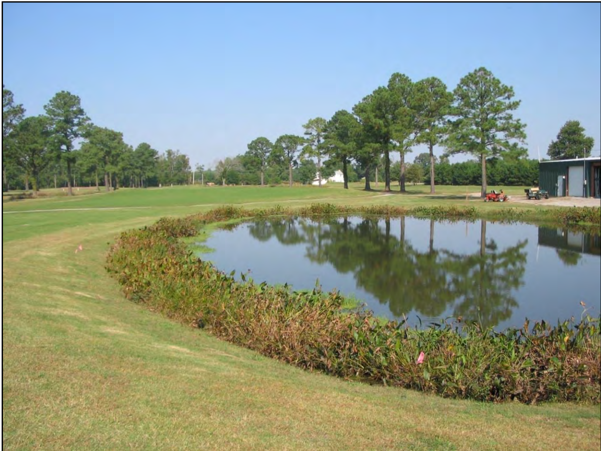
Figure B-12: Example of a Wet Detention Basin with Vegetated Shelf (NCSU BAE, 2011)
