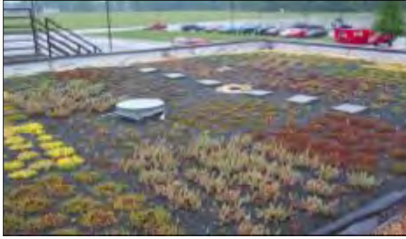
Figure B-31: Example of Extensive Green Roof (New Hanover County & City of Wilmington, 2008)
