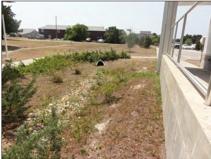
Figure 2-6: Example of a Stormwater Swale
