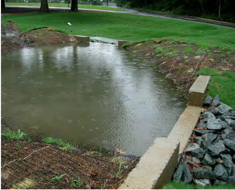
Figure B-2: Example of a Forebay (NCSU, 2009)
