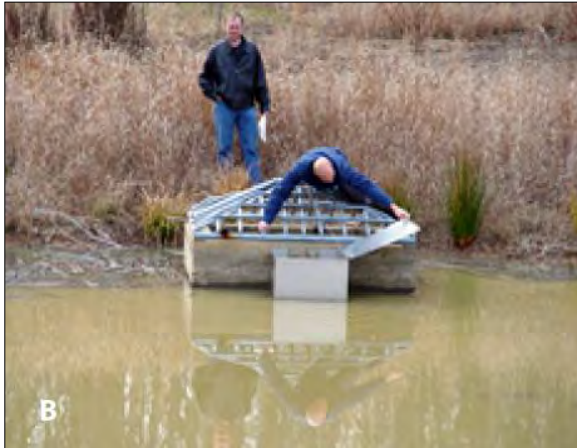
Figure B-11: Example of a Trash Rack (Hunt, Burchell, Wright, & Bass, 2007)
