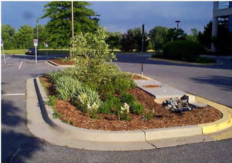
Figure B-21: Bioretention Cell in Parking Lot Island (NCDWQ, 2007)
