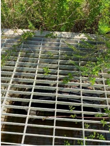
33. Pond 2 outlet control structure.
