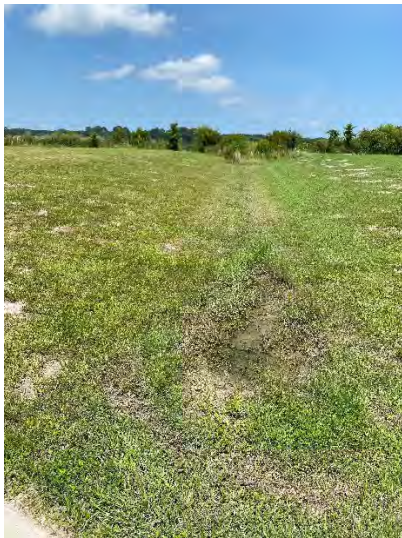
41. Typical collector swale.
