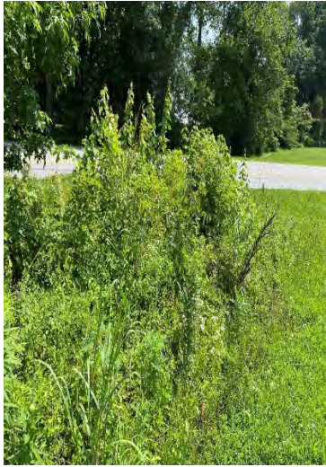
38. Overgrown outlet ditch from Pond 2
