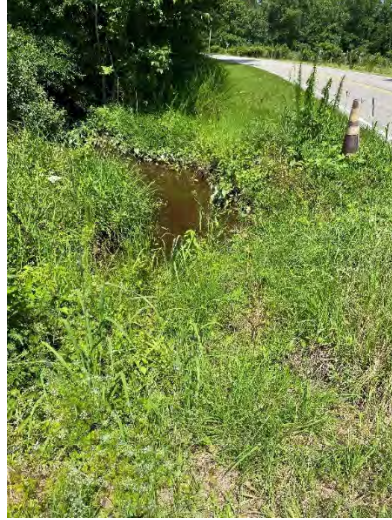
40. Pond 2 outlet ditch at Guinea Road culvert entrance.
