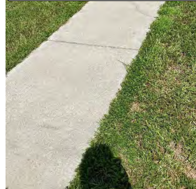
12. Sidewalk sections along side of Phase 1 pond needs repair
