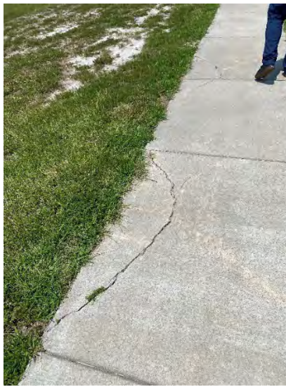
12. Sidewalk sections along side of Phase 1 pond needs repair
