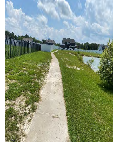
10. Sidewalk along east side of Phase 1 pond.
