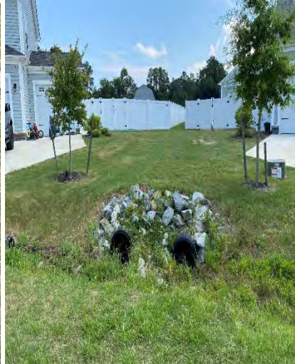
45. Twin culvert entrance on Gables Place.
