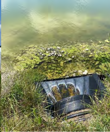
28. Culvert entering Phase 1 pond.
