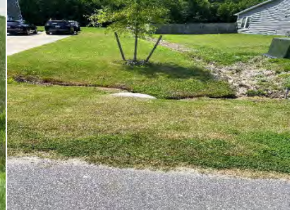
46. Swale and culvert at lots 15 & 16 on Gables Place.
