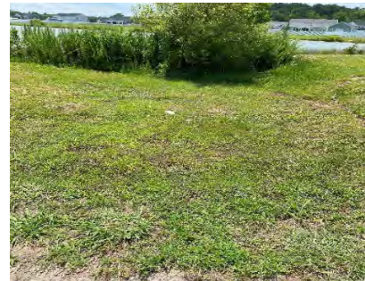
49. Vegetated collector ditch entering Pond 1 from northeast.
