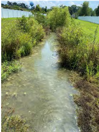
35. Outlet ditch from Pond 1.
