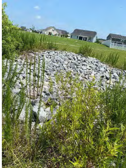
42. Riprap protection at inlet to Pond 1 from the northeast.
