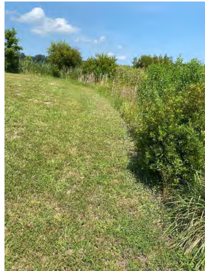
43. Vegetation protecting overflow ditch from northeast (Note: Due to past problems with erosion in this area, it is recommended that woody vegetation remain.)
