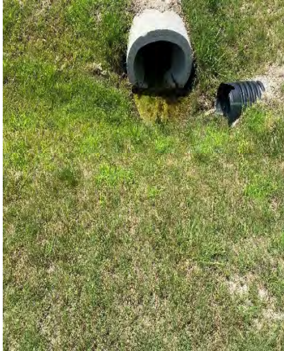
44. Culvert near lots 24 & 25.
