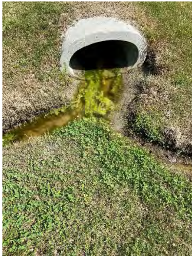
47. Closeup of culvert entrance (pipe is clear).
