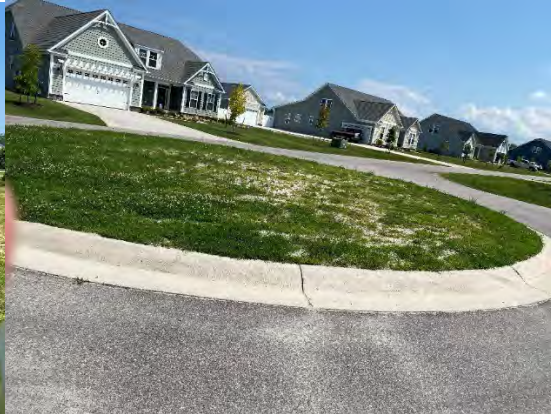
56. Cul-de-sac at end of Briton Way (association maintenance responsibility).
