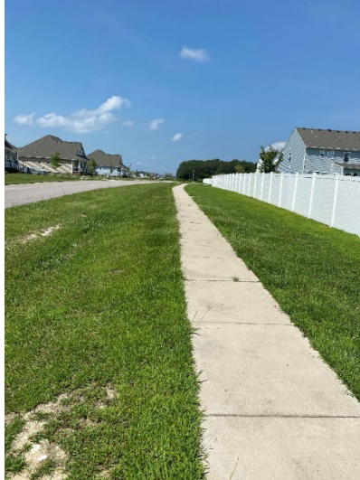
18. Sidewalk along Thayne Drive.
