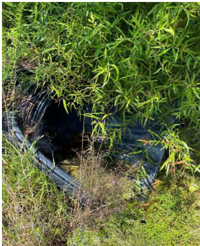
30. Culvert inlet to Phase 1 by Gables Place (needs minor vegetation removal).
