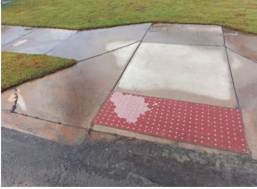
Photo #18 - Pedestrian Crossing in front of Lot 15, Facing North
