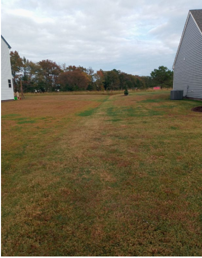
Photo #47 - Swale between Lot 50 and Lot 51, Facing East
