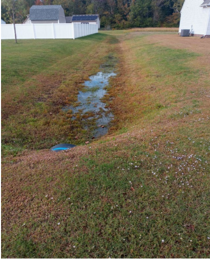
Photo #44 - Swale on West side of Lot 9, Facing North
