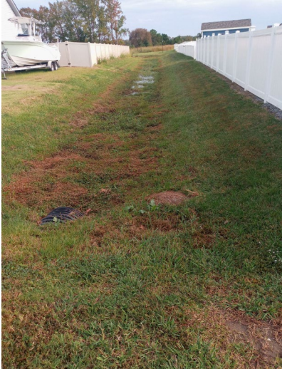
Photo #48 - Swale on West side of Lot 45, Facing Southeast
