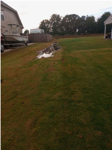
Photo #45 - Outgoing Swale between Lot 2 and Lot 3, Facing West
