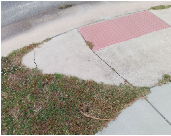
Photo #34 - Pedestrian Crossing on the North side of Lot 15, Facing Southwest
