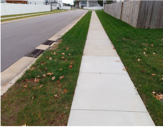
Photo #3 - Sidewalk between Lot 56 and Lot 57, Facing West
