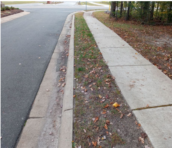
Photo #13 - Sidewalk on the South side of the Entrance, Facing East
