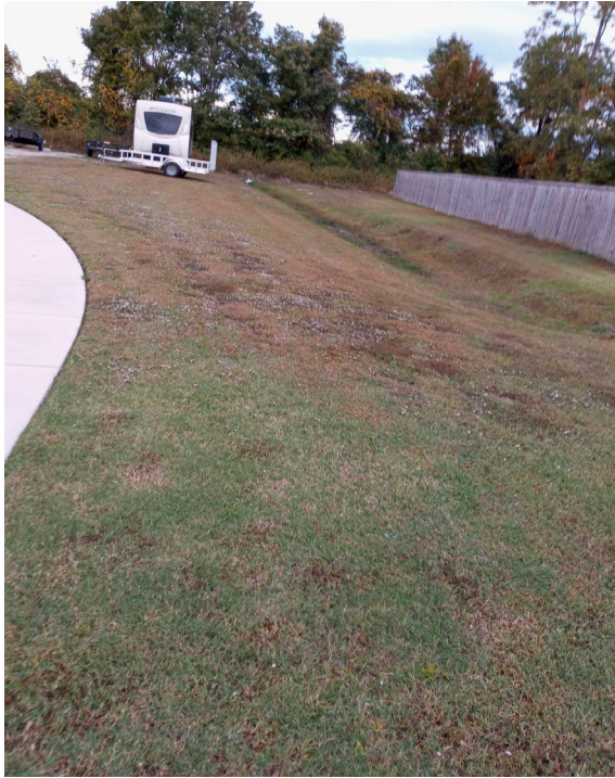
Photo #64 - Swale between Lot 1 and RV/Trailer Parking, Facing North
