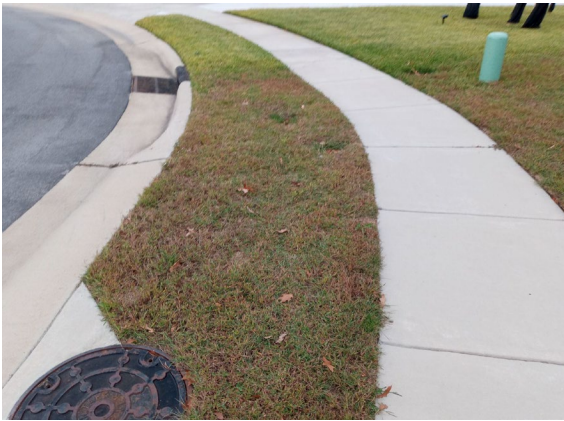
Photo #20 - Sidewalk between Lot 12 and Lot 13, Facing West
