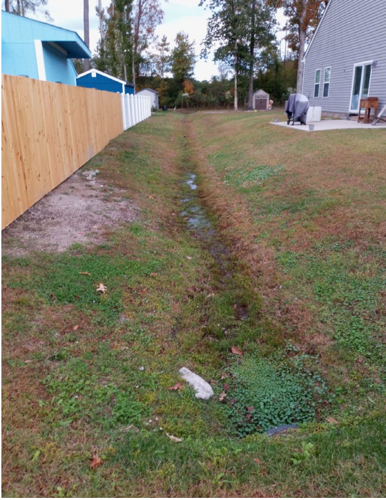
Photo #63 - Swale between Lot 8 and Lot 9, Facing North has some extra vegetation that should be cut
