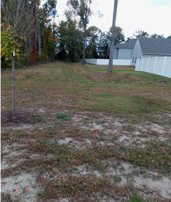
Photo #57 - Swale between lot 57 and Lot 58, Facing South
