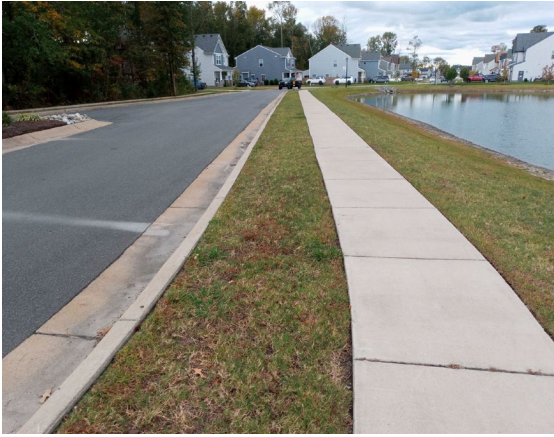
Photo #14 - Sidewalk on the North side of the Entrance, Facing West
