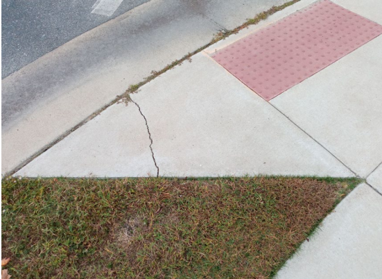
Photo #31 - Pedestrian Crossing on the Southeast side of Lot 22, Facing Southwest
