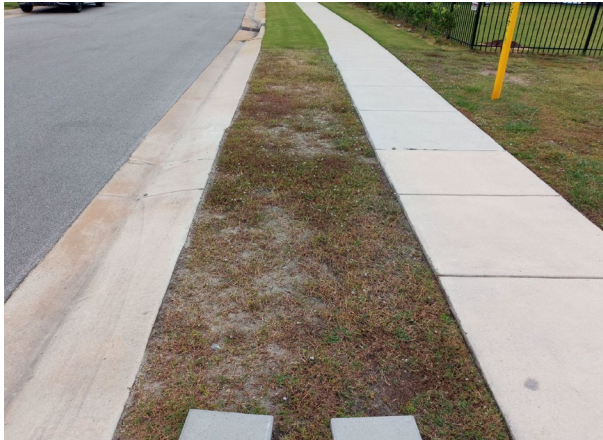
Photo #1 - Sidewalk on North side of Lot 67, Facing East
