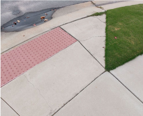
Photo #37 - Pedestrian Crossing on the West side of Lot 9, Facing South
