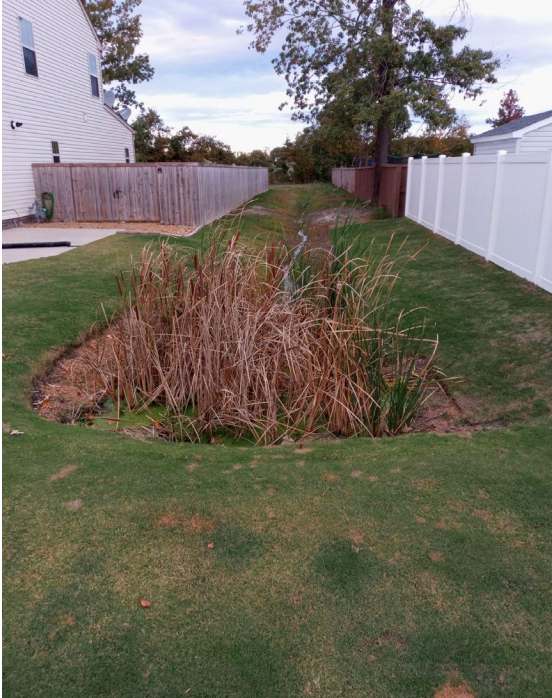
Photo #63 - Swale between Lot 8 and Lot 9, Facing North has some extra vegetation that should be cut
