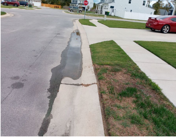
Photo #4 - Sidewalk in front of Lot 48, Facing North
