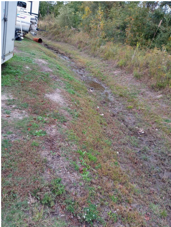
Photo #65 - West side of Swale behind Trailer Parking, Facing West
