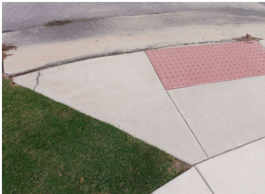
Photo #27 - West side of the Pedestrian Crossing on Lot 48, Facing North
