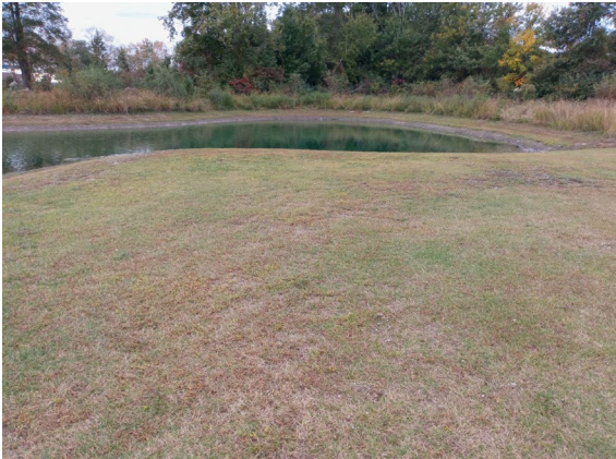
Photo #44 - North side of Stormwater BMP 2, Facing Northwest
