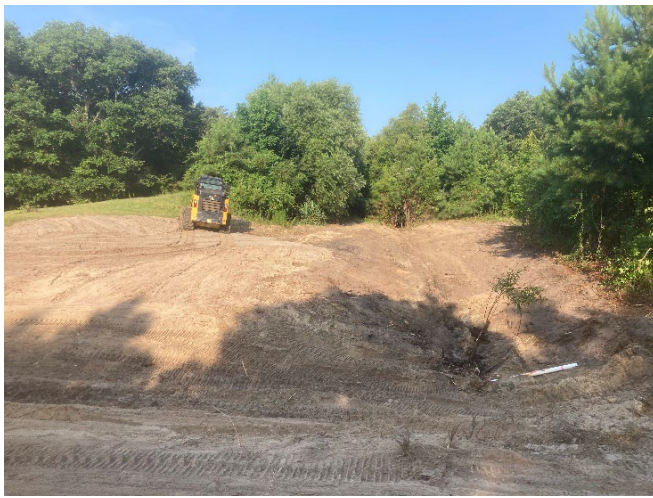
Another view of roadway and swale repair.
