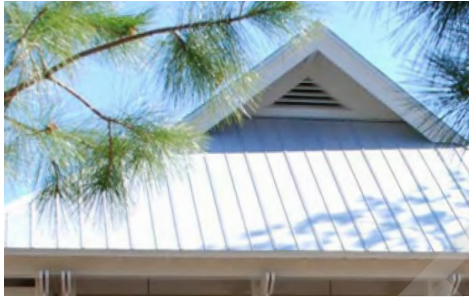
Standing seam metal. 1 1/2" vertical seam with 12"-18" spacing. Silver metallic, medium gray, dark green, or dark red in color
