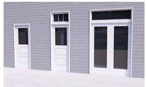
Doors and windows set in cedar or cypress shake siding with 1 1/2" to 3" flat trim.
