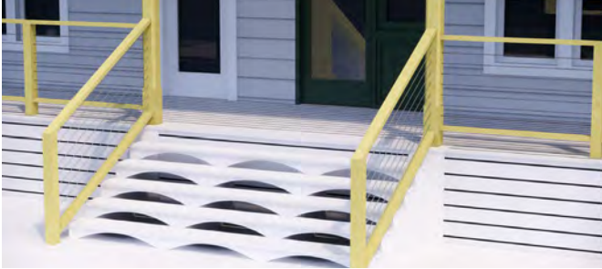
Cable Railing Contemporary style of railing with high visibility and horizontal emphasis
