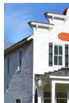
Wood or fiber cement clapboard siding in a variety of colors in whites, grays, earth tones, and pastels are appropriate. Exposures should be 8" or less.
