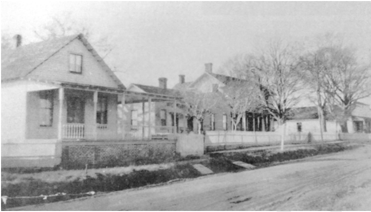
Courthouse Road, Currituck, NC
