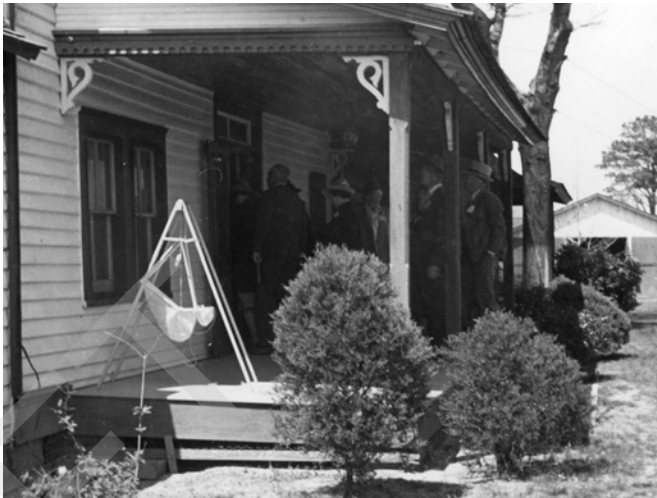
Vernacular porch with decorative brackets and trim
