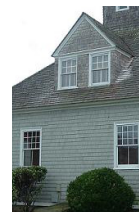
Cedar shake or fiber cement simulated shake siding, stained, painted, or natural, is appropriate. Colors should be whites, grays, earth tones, or pastels.
