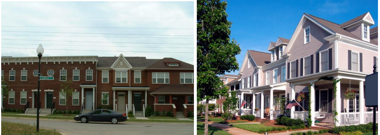
Figure 5.7.3.C, Front Facades and Roof Forms
