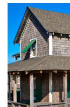
Cedar shake or fiber cement simulated shake siding, stained, painted, or natural, is appropriate. Colors should be whites, grays, earth tones, or pastels.
