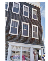
Cedar shake or fiber cement simulated shake siding, stained, painted, or natural, is appropriate. Colors should be whites, grays, earth tones, or pastels.
