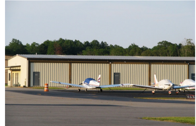
Currituck County Airport The recently added hangers at Currituck Airport.
