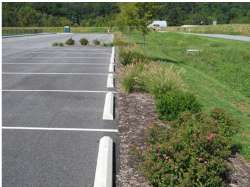
Figure 5.1.4.11, Parking Lot Stormwater Devices
