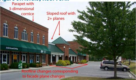
(c) When flat roofs are used, parapet walls with three-dimensional cornice treatments shall conceal them. The cornice shall include a perpendicular projection a minimum of eight inches from the parapet façade plane.
