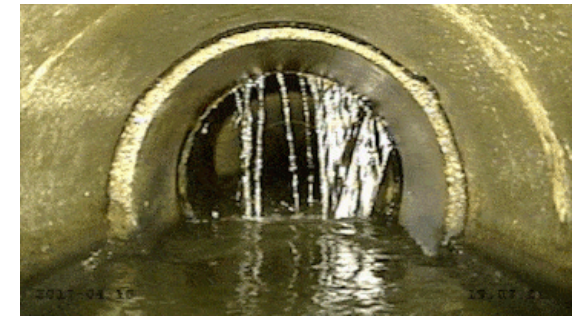
Example of Infiltration source - Inside view of water coming into sanitary sewer pipe
