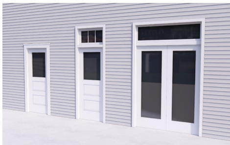
Doors and windows set in clapboard siding with trim 3" to 6" in width. The door/window trim width should always be less than the width of the corner trim of the building.
