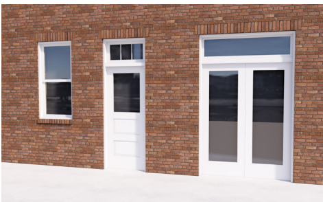
Doors and windows set in brick - recessed with brick mold with brick lintels or arches above and brick or wood/composite sills below.
