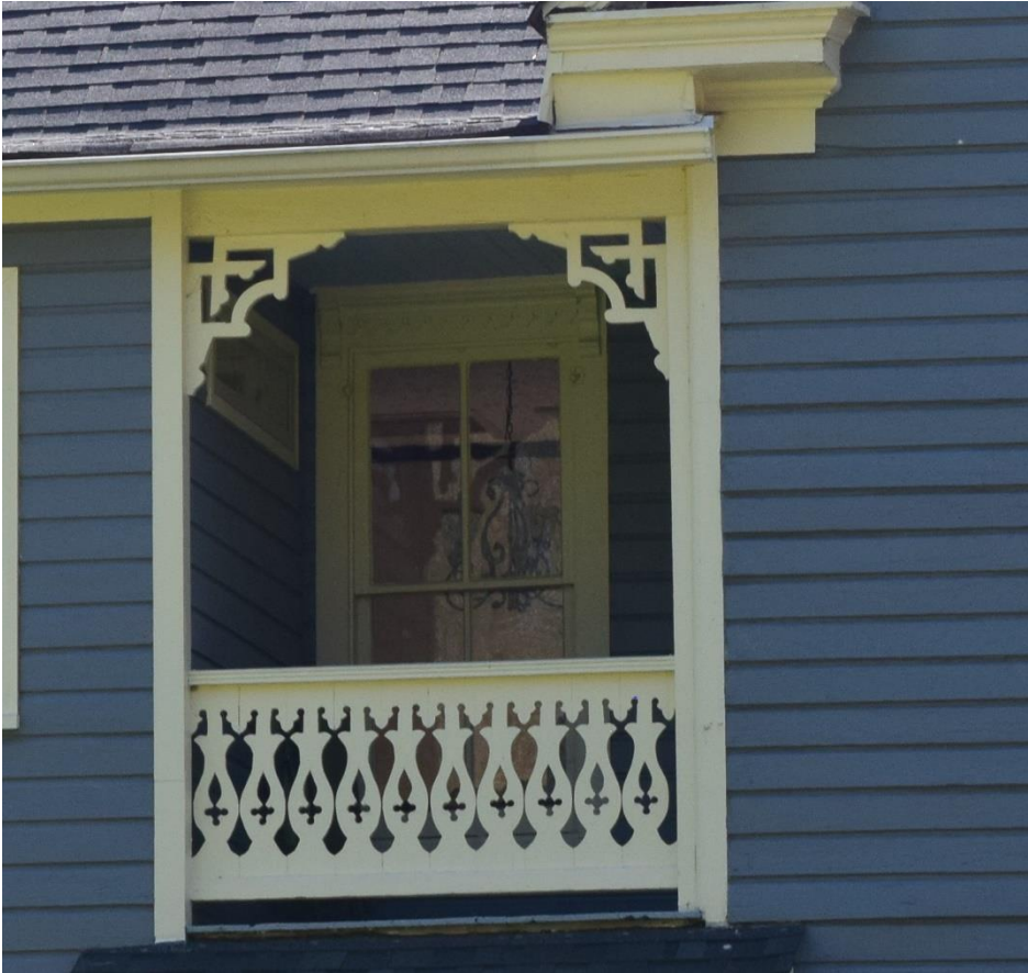
Fig. 20: Balustrade and Bracket Detail
