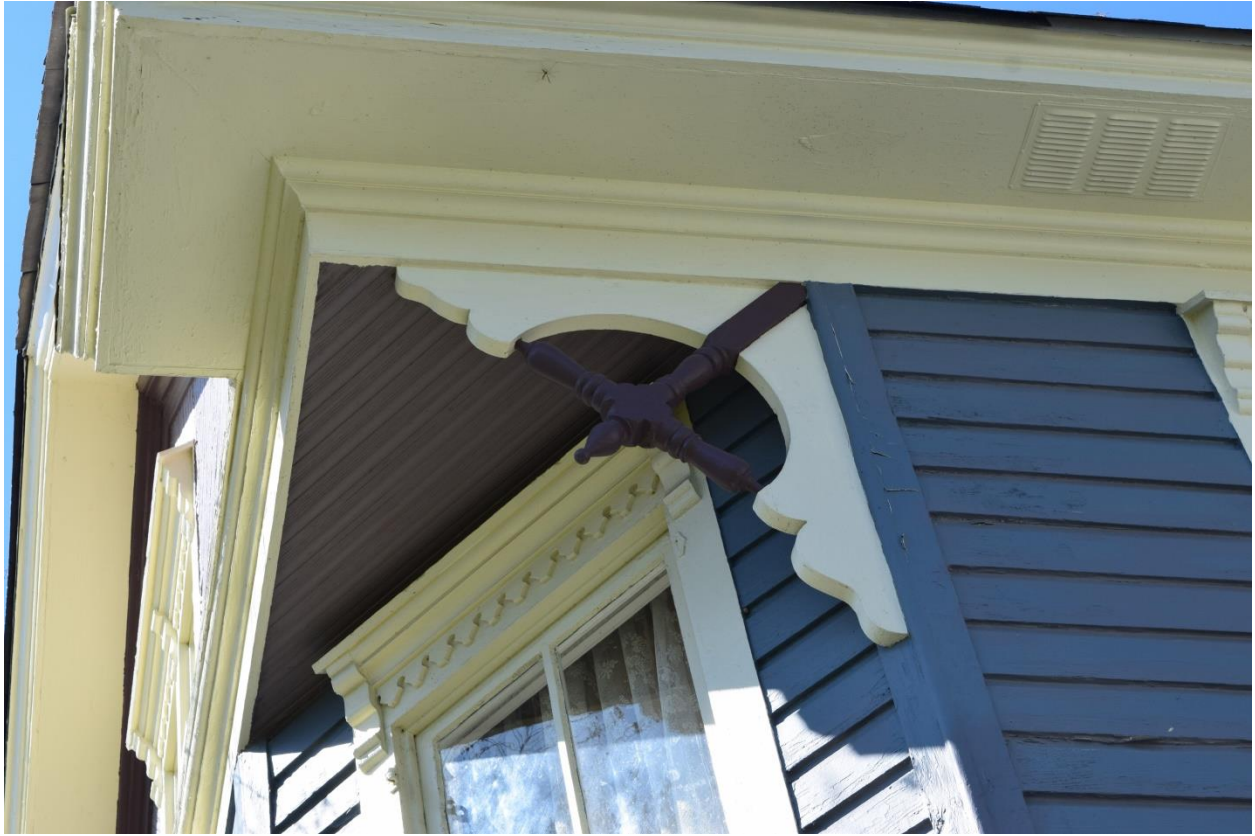
Fig. 4: Bracket under Front Gable
