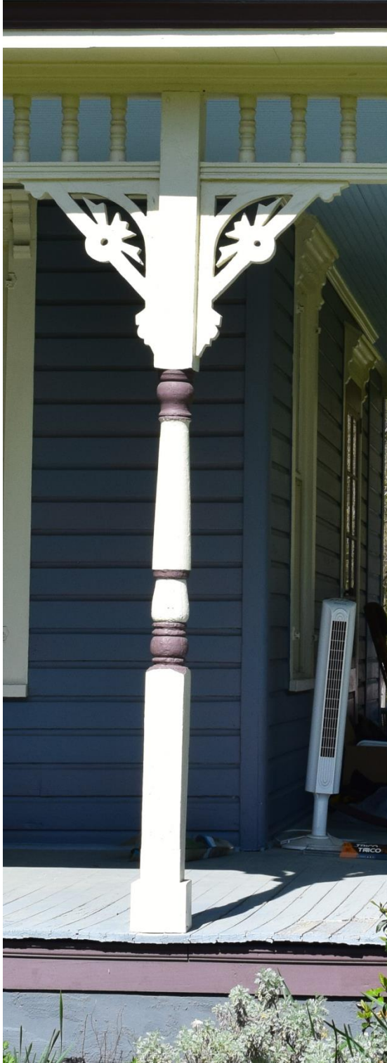
Fig. 8: Turned Porch Spindles, Porch Floor and Trim
