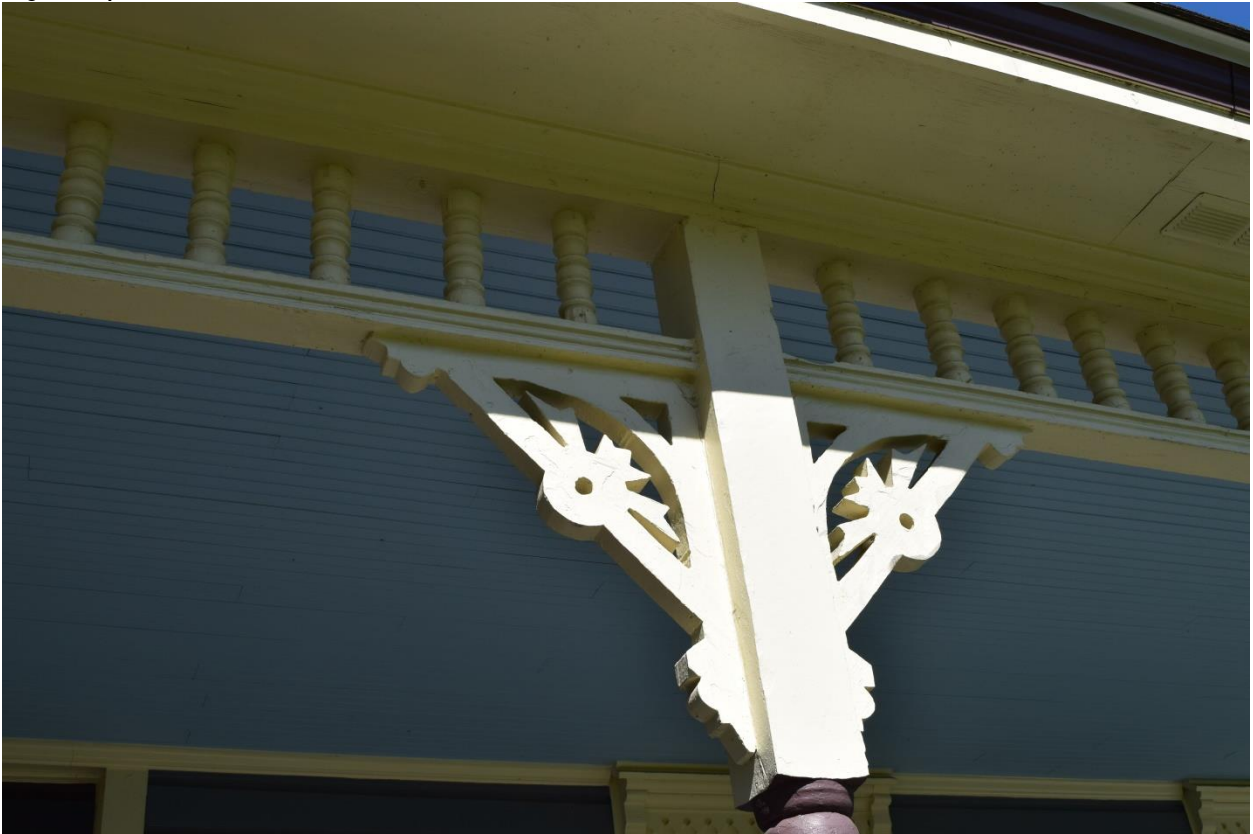
Fig. 7: Spindle Frieze and Brackets
