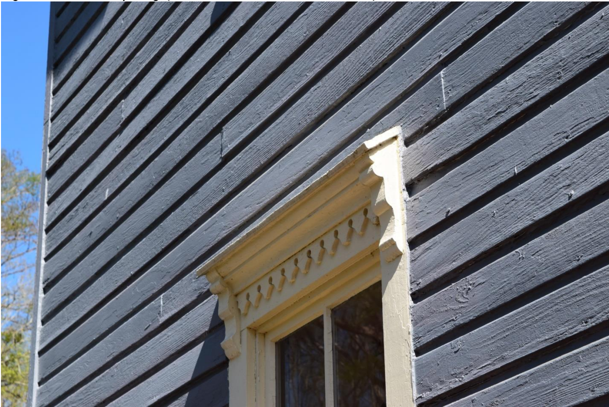
Fig. 10: Molded drip edge, sawtooth ornament and scrolled, console like brackets
