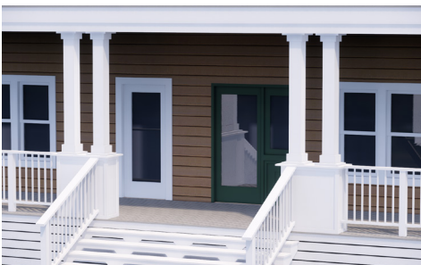
Double Columns on plinths Contemporary style. Plinths can be wood or masonry
