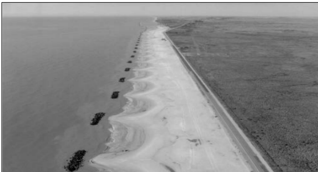
Figure 90. Example of a breakwater field and a renourished beach at Holly Beach, Louisiana (Mann and Thomson, 2003)
