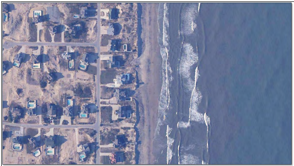
Figure 13. Post Hurricane Isabel Imagery showing severe scarping and dune washout along the Ocean Hills Community following Hurricane Isabel (2003). Source: National Geodetic Survey - Emergency Response Imagery Index .
