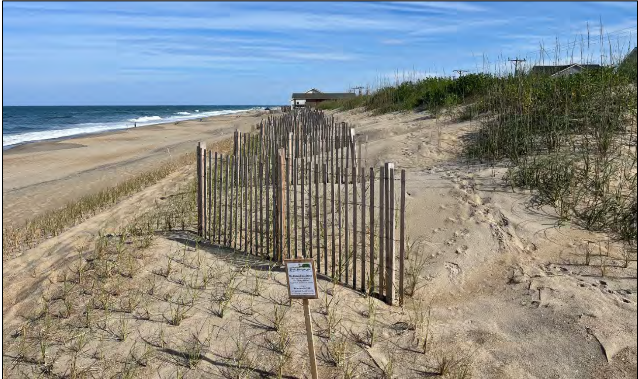
Figure 91. A constructed dune in the Town of Kitty Hawk, NC where dune vegetation was planted along the seaward dune slope and crest and sand fence was installed along the crest (May, 2023).
