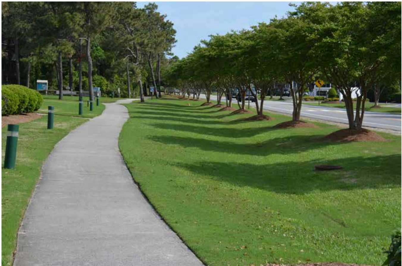
The Corolla Greenway is an example of a trail separated far from the roadway for increased pedestrian comfort.
