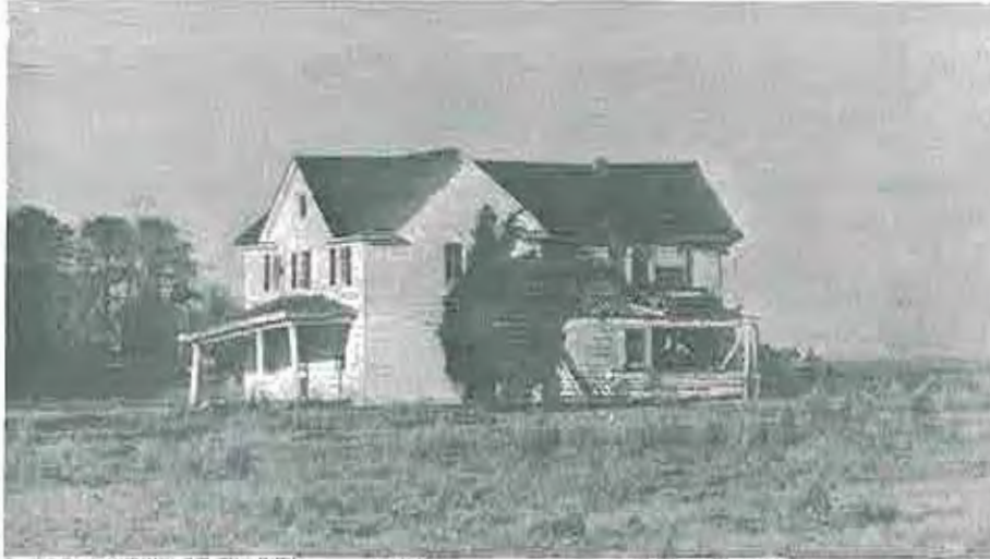
Dilapidated buildings detract from appearance
