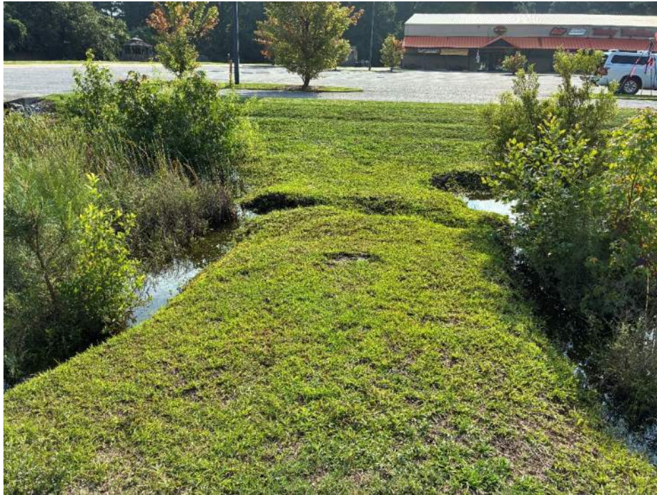
Photo 9 – View of forebay berm from the east.
