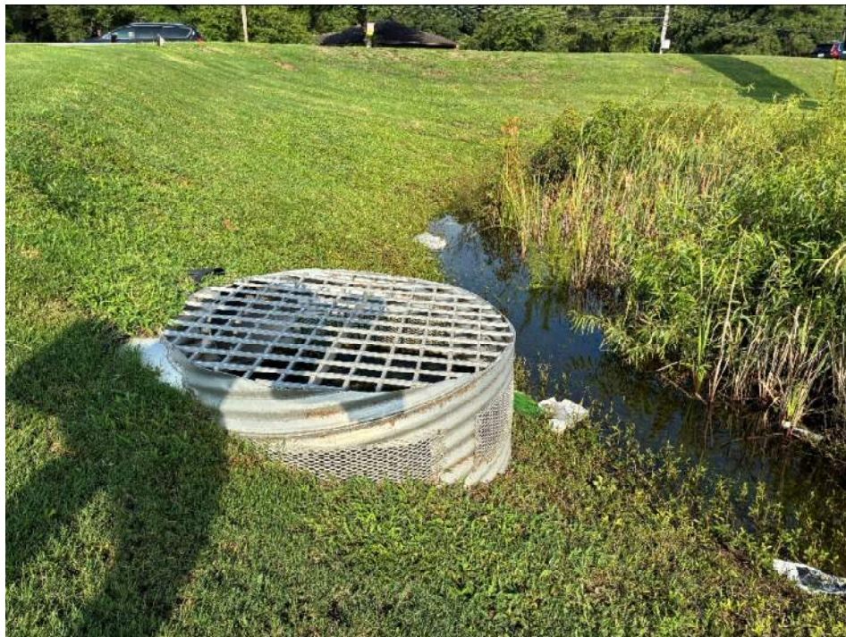
Photo 12 – Overflow device on the south side of the forebay.
