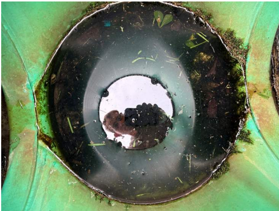
Photo 18 – Typical view within drop inlets.
