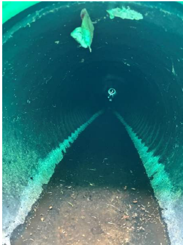
Photo 20 – Typical view within culvert pipes beneath drop inlets.
