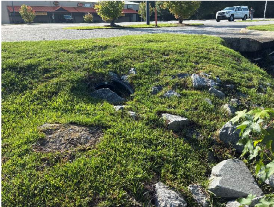
Photo 5 – Culvert inlet from the east drop inlets draining into the main treatment area.
