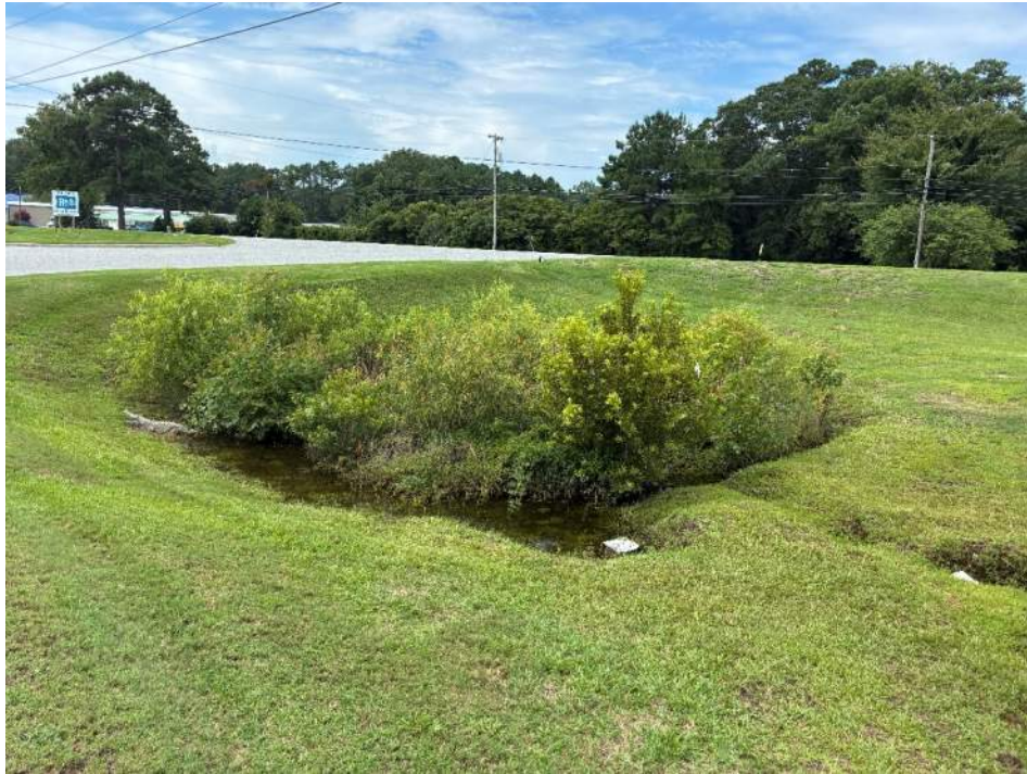
Photo 11 – View of the forebay from the east.
