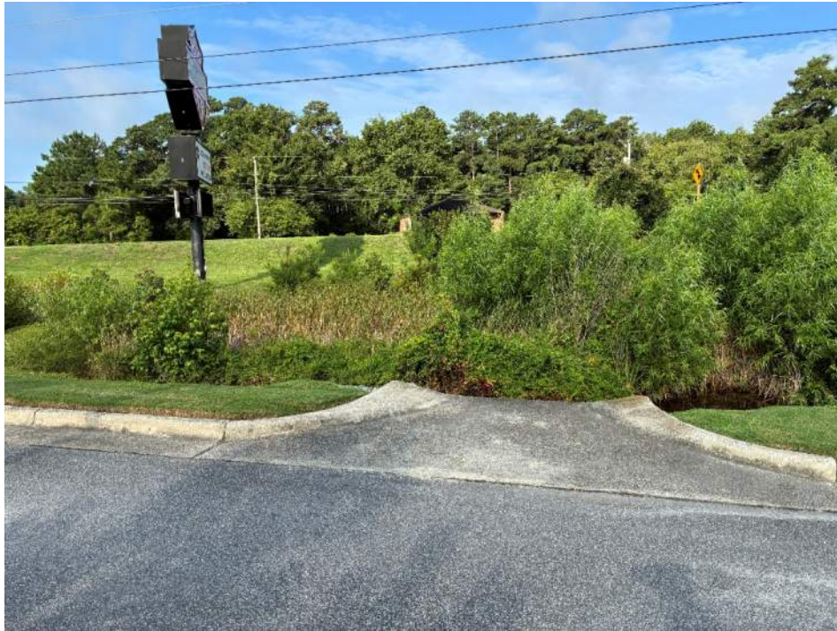
Photo 7 – View of concrete flume along the east side of the retention pond.
