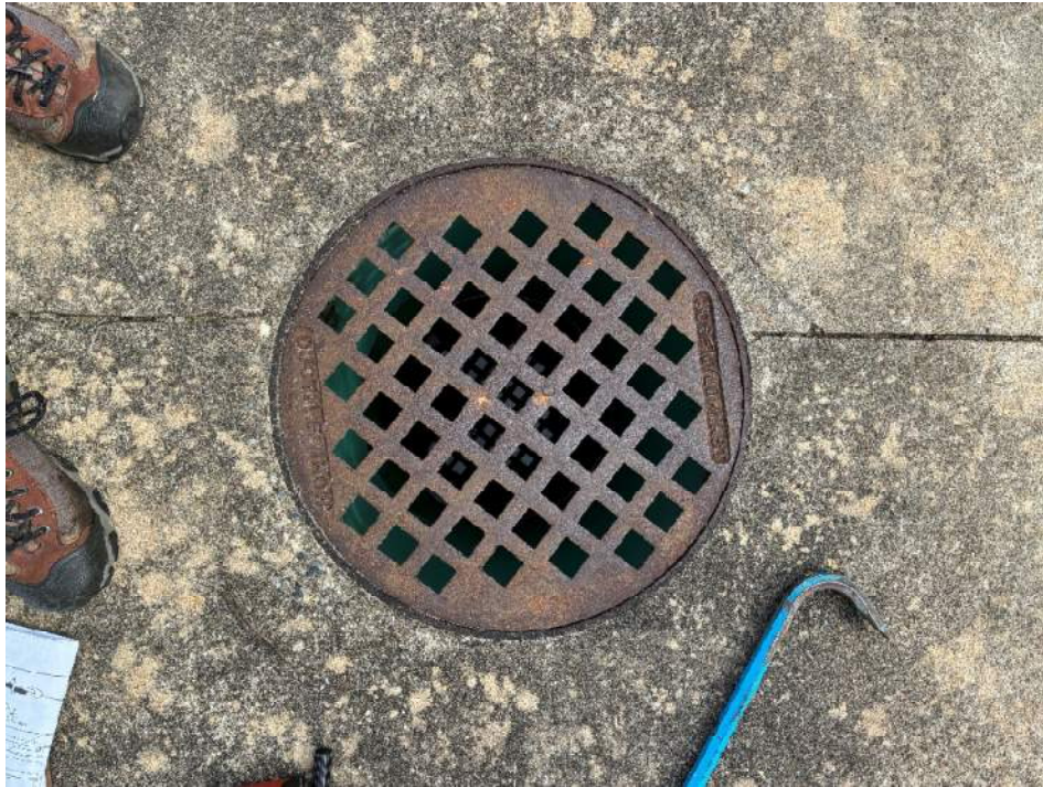
Photo 19 – Easternmost drop inlet east of the main treatment area.
