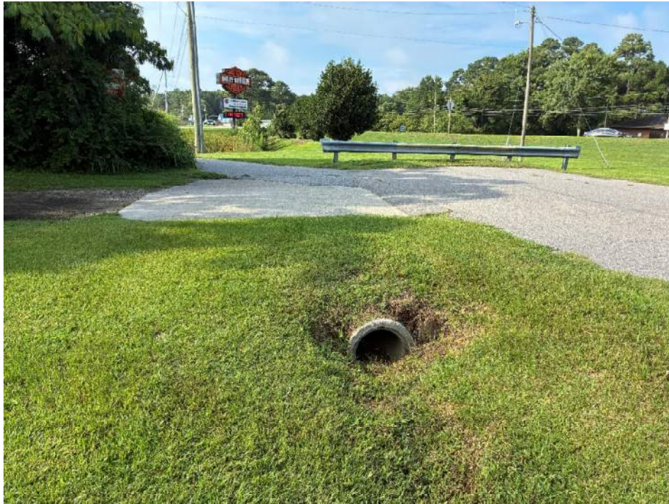
Photo 3 – North end of the culvert seen in Photo 2.
