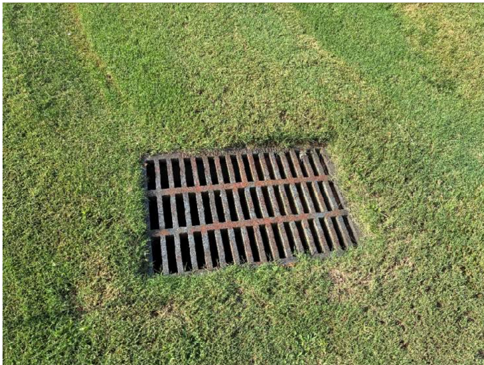
Photo 14 – Drop inlet south of the overflow device.
