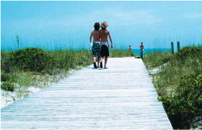
Photo 18: This is an on-grade walkway without railings.
