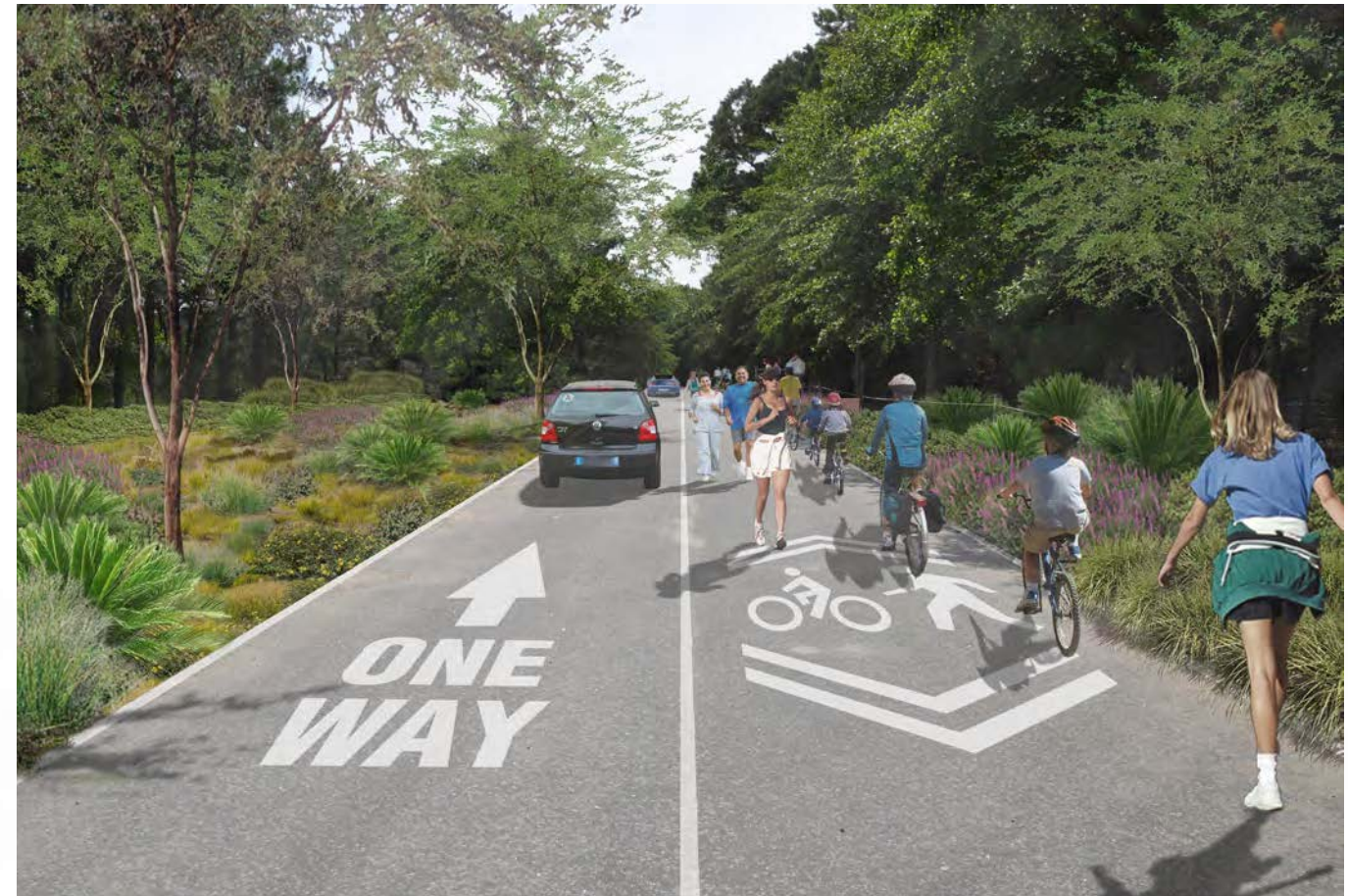
The first phase of the one-way conversion employs precedents set by Duck and Nags Head in the Outer Banks. Striping will provide separation within the roadway for pedestrians and cyclists. Parking will remain on the south side of Corolla Village Road.
