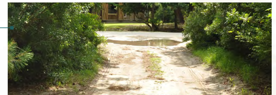
Conditions are not suitable on some roads (Carotank Drive) for encouraging bicycle circulation.
