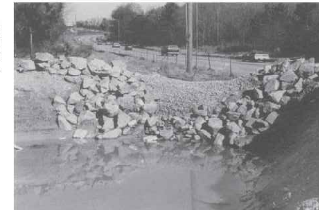
Figure 6.60 Temporary settling pool traps sediment.
