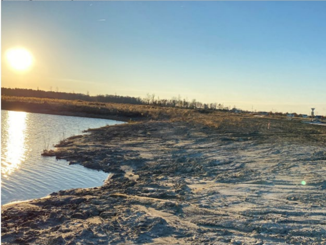
Picture 5) Pond 3 has a bit of erosion affecting the shelf. Not part of this phasing, but still please note.
