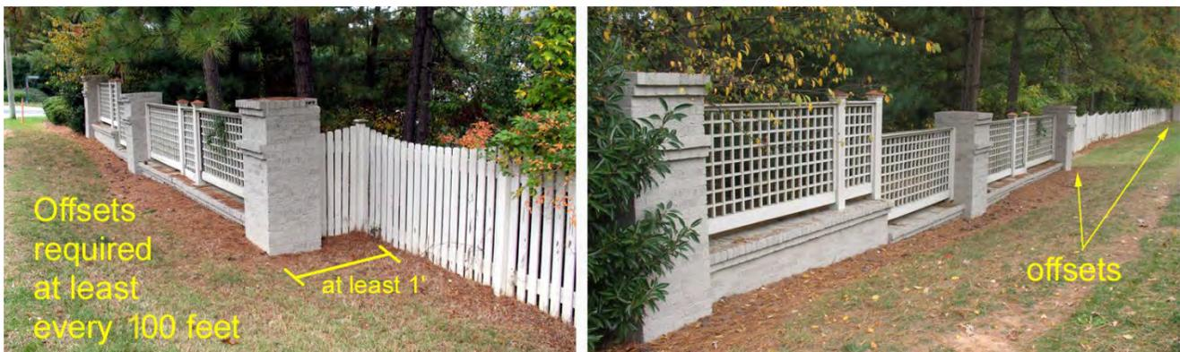
Figure 5.3.6.A, Design Features for Opaque Fences and Walls
