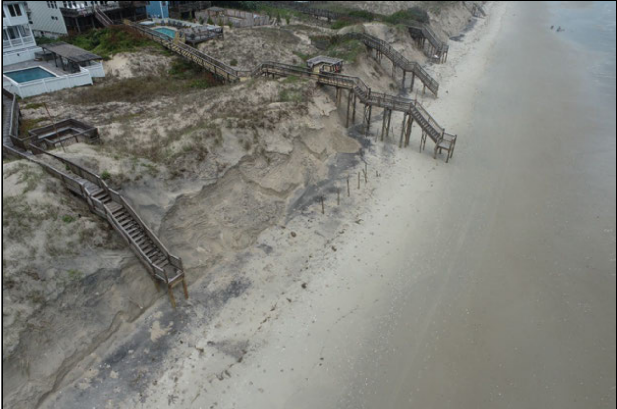
Figure 20. View of Dune Scarping approximately 500 feet north of Sta. C-060. (Photo date 5/15/22).
