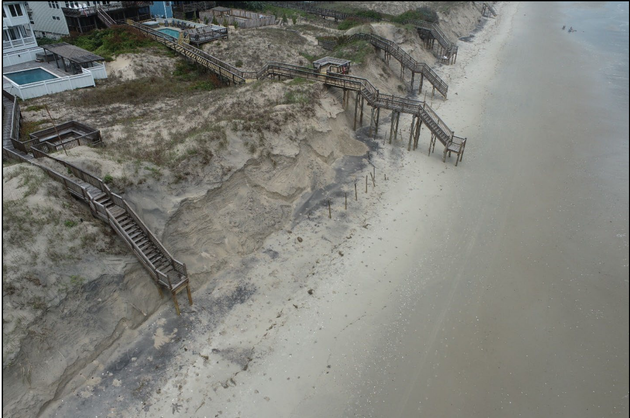
Figure 24. View of Dune Scarping approximately 500 feet north of Sta. C-060. (Photo date 5/15/22).
