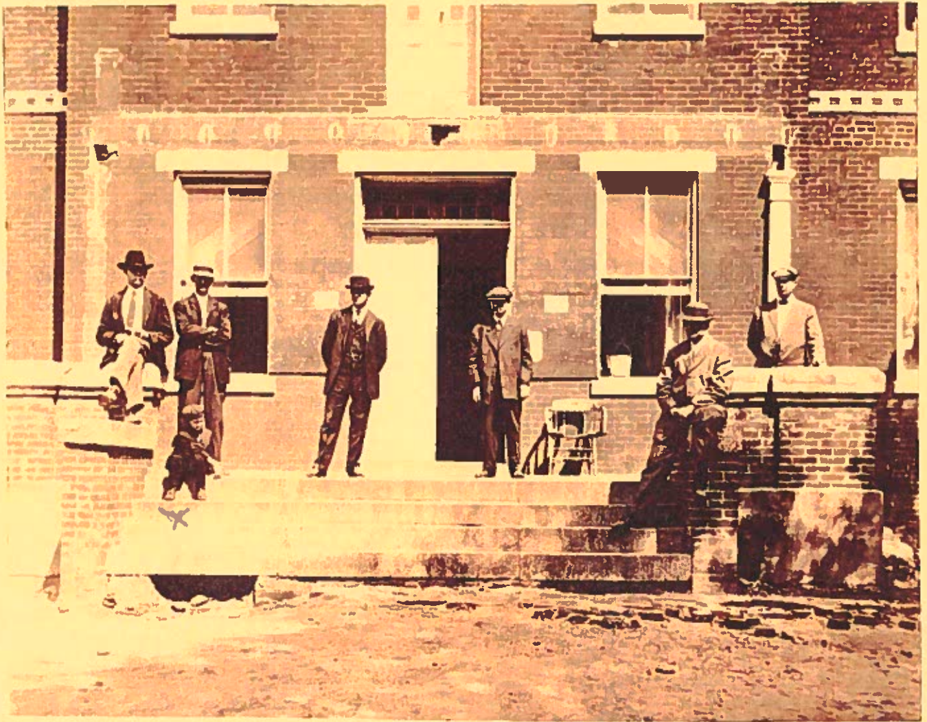
Figure 10. Currituck County Courthouse after dismantling of front porch, c. 1910-1920. Collection of Mrs. Barbara Snowden, Currituck, N.C.
