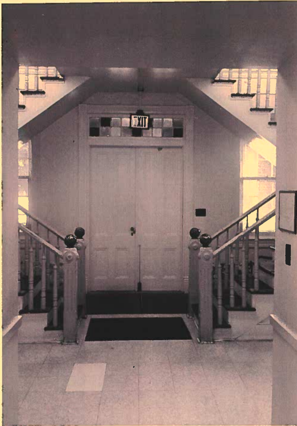
Figure 40. Currituck County Courthouse, entrance hall, front door and double stair, 1897-1898.
