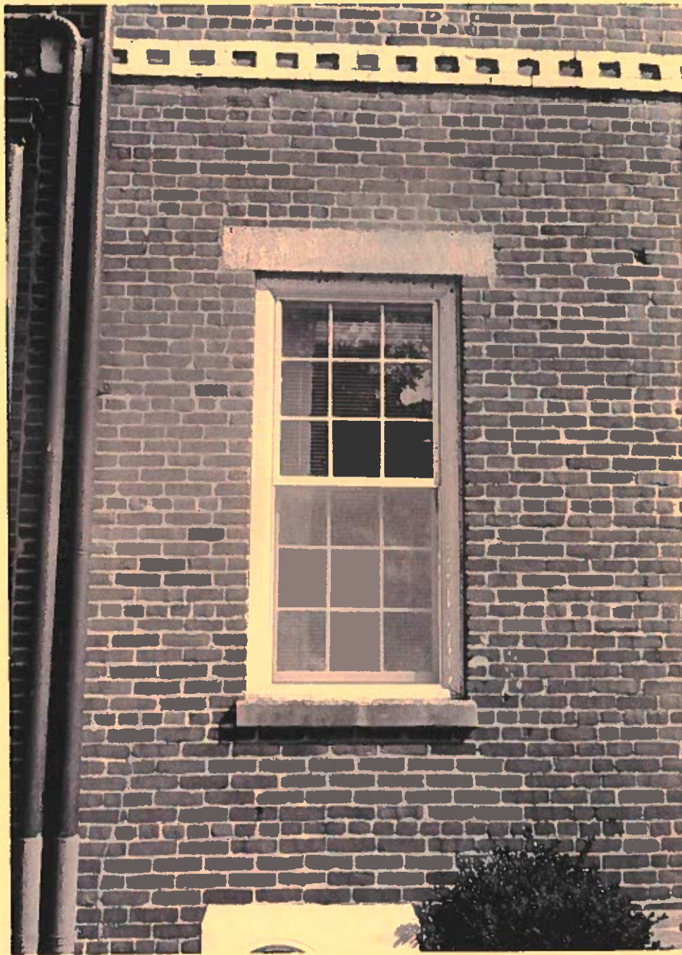
Figure 32. Currituck County Courthouse, window, west elevation, first-story, 1897-1898. [ replacement sash ]
