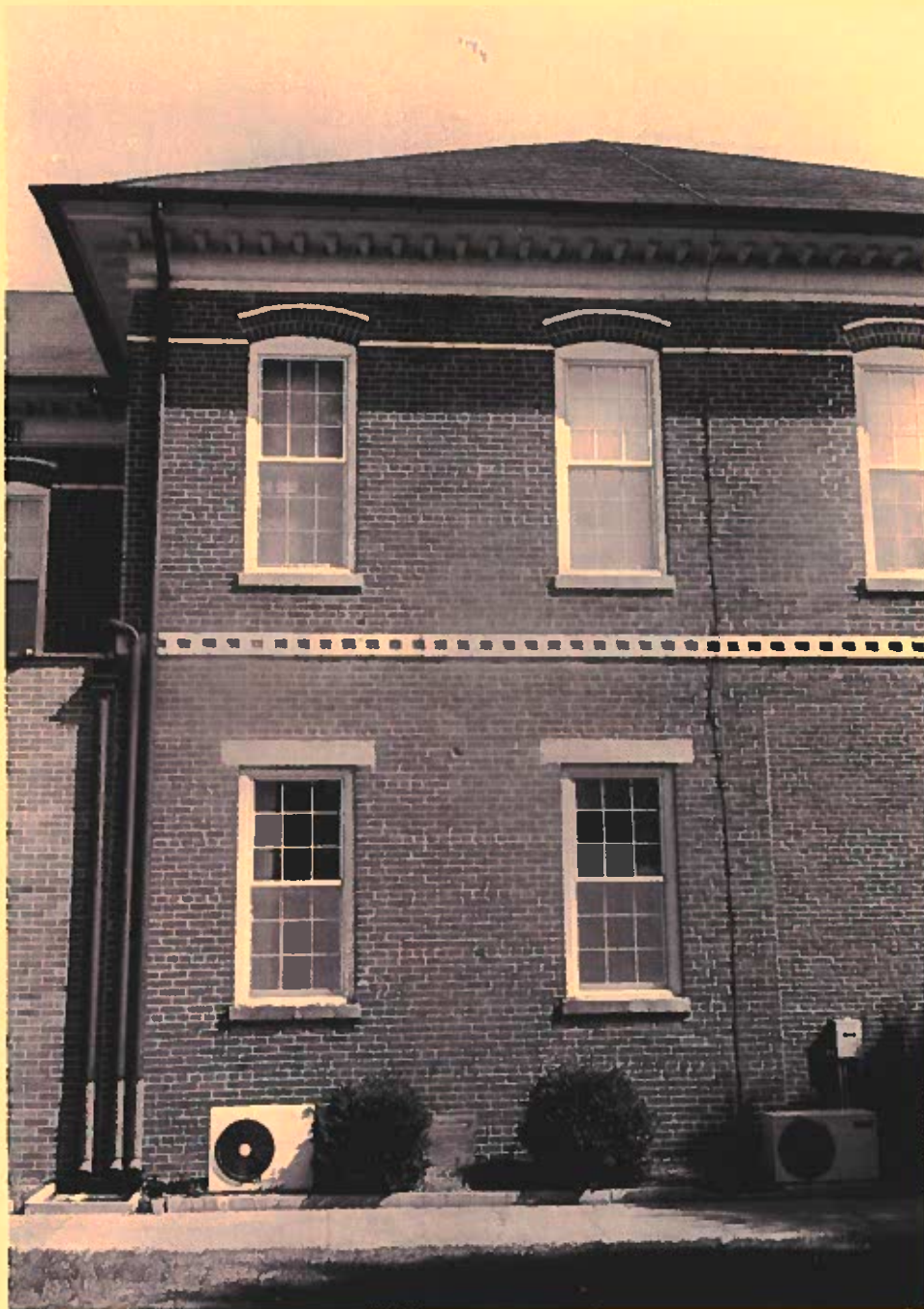
Figure 31. Currituck County Courthouse, west elevation, 1897-1898 addition.
